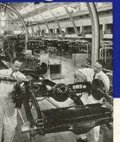
Much of the chassis is assembled upside down. After the springs and other parts are in place, the rear axle swings into place on an overhead hoist. Chevrolet workmen rapidly fasten the axle to the rear springs and tighten up the bolts which hold it in place. The new Y-K frame for 1934 is 15 times stronger than conventional
