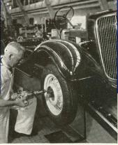
Familiar operations — mounting the tires on the wheels and then putting the wheels on the car. Running boards, with the front and rear fenders, are assembled at the side, then added to the chassis. Meanwhile, workmen on the end of the Fisher Body line are installing the instrument panel, electric wiring, lights and switches.
