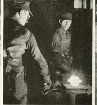
A few seconds after this photograph was taken, the glowing mass of metal had been formed into two front wheel spindles for Knee-Action units, and a similar white-hot lump of steel was ready to be placed under the
