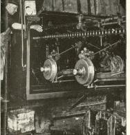
Complete front-end units are taken from the end of the conveyor assembly line and travel through a tunnel, suspended from an overhead conveyor. In this tunnel, a lacquer finish is sprayed on the metal.
