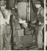
A billet of glowing hot steel, nearly shapeless, is placed under the steam hammer, and with a few blows between the dies the desired shape is formed. The Chevrolet forge shop is the largest in the world, in the number of hammers and in output tonnage.
