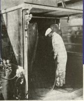
First Chevrolet operation. Fenders, hoods and other parts are rubbed smooth with sandpaper, rubbed smooth with sandpaper, then taken to a glass booth. Four coats of Duco are applied with spray guns, and the parts are hung on racks to dry. In another glass booth, Duco is applied to the radiator shell and other parts, the wheels being coated with Dulux enamel.
